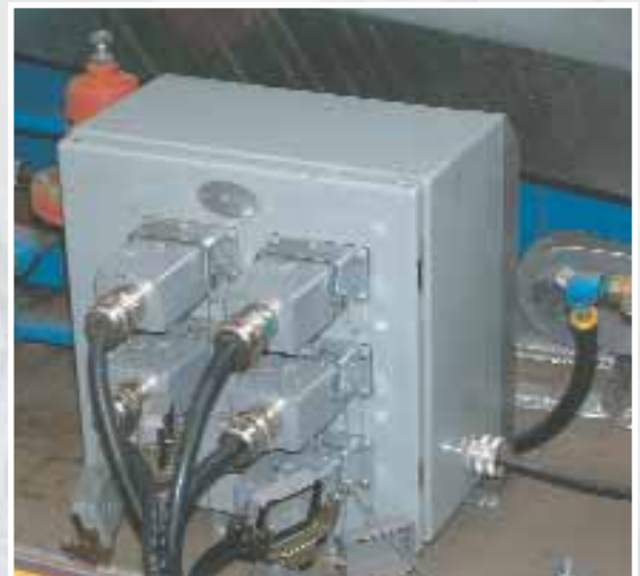
All electrical connections are designed to withstand extremes of temperature and the rigors of on-site conditions. This set of connectors integrates the feed system motors with main processing unit.
